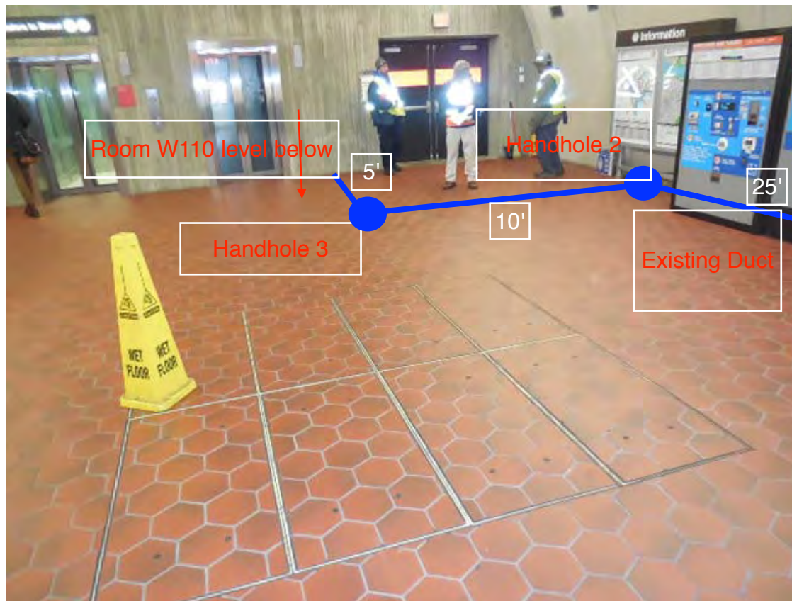
Photo 2 – Existing duct layout on mezzanine floor.
